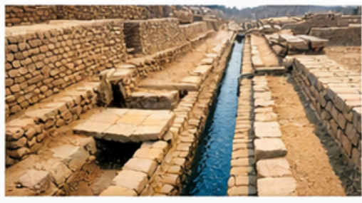
Well-Planned Drainage System
