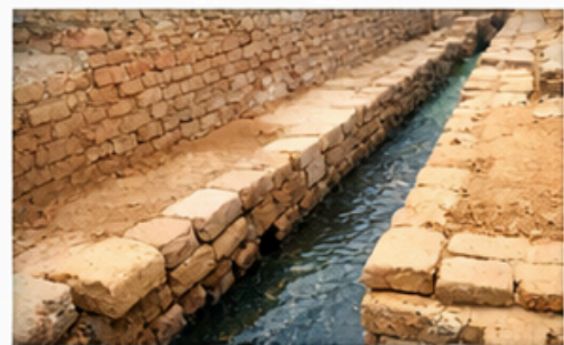
Cesspits Carry Dirty Water Outside
